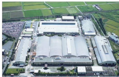
MITSUBISHI MATERIALS AKASHI PLANT (JAPAN)
